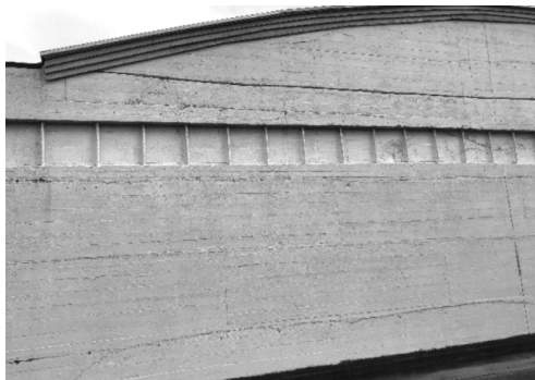
Exterior West wall of Gymnasium.
